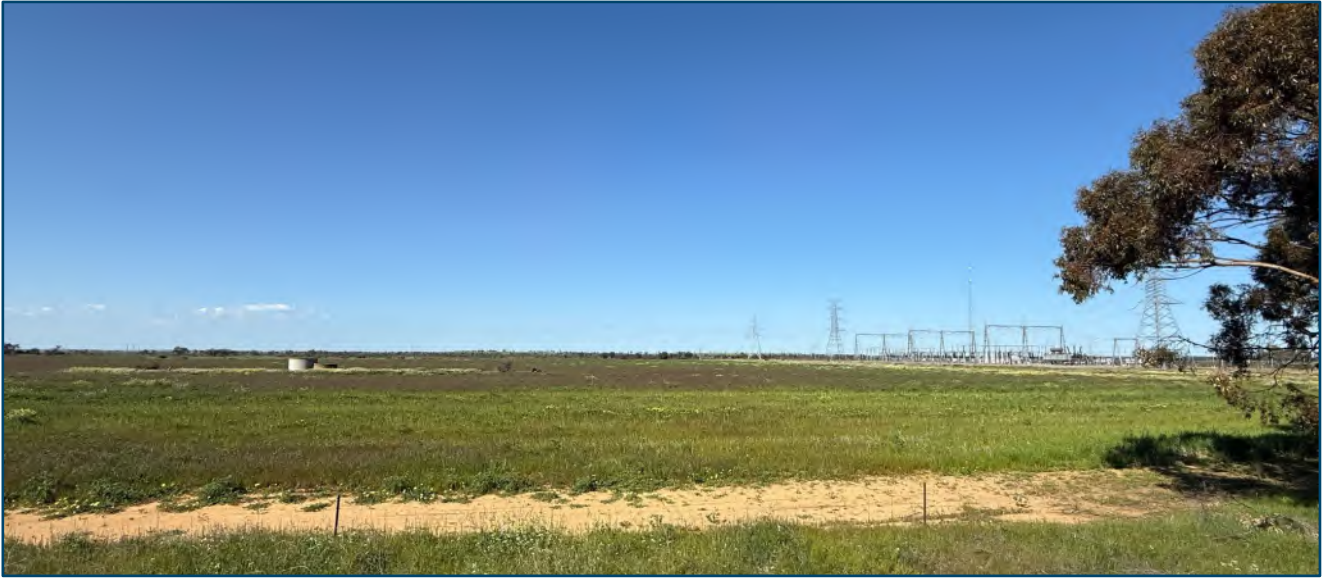
Figure 4 – Site photograph of Lot 25 and the Western Power substation (Lot 22), looking south from Perenjori-Three Springs Road.
