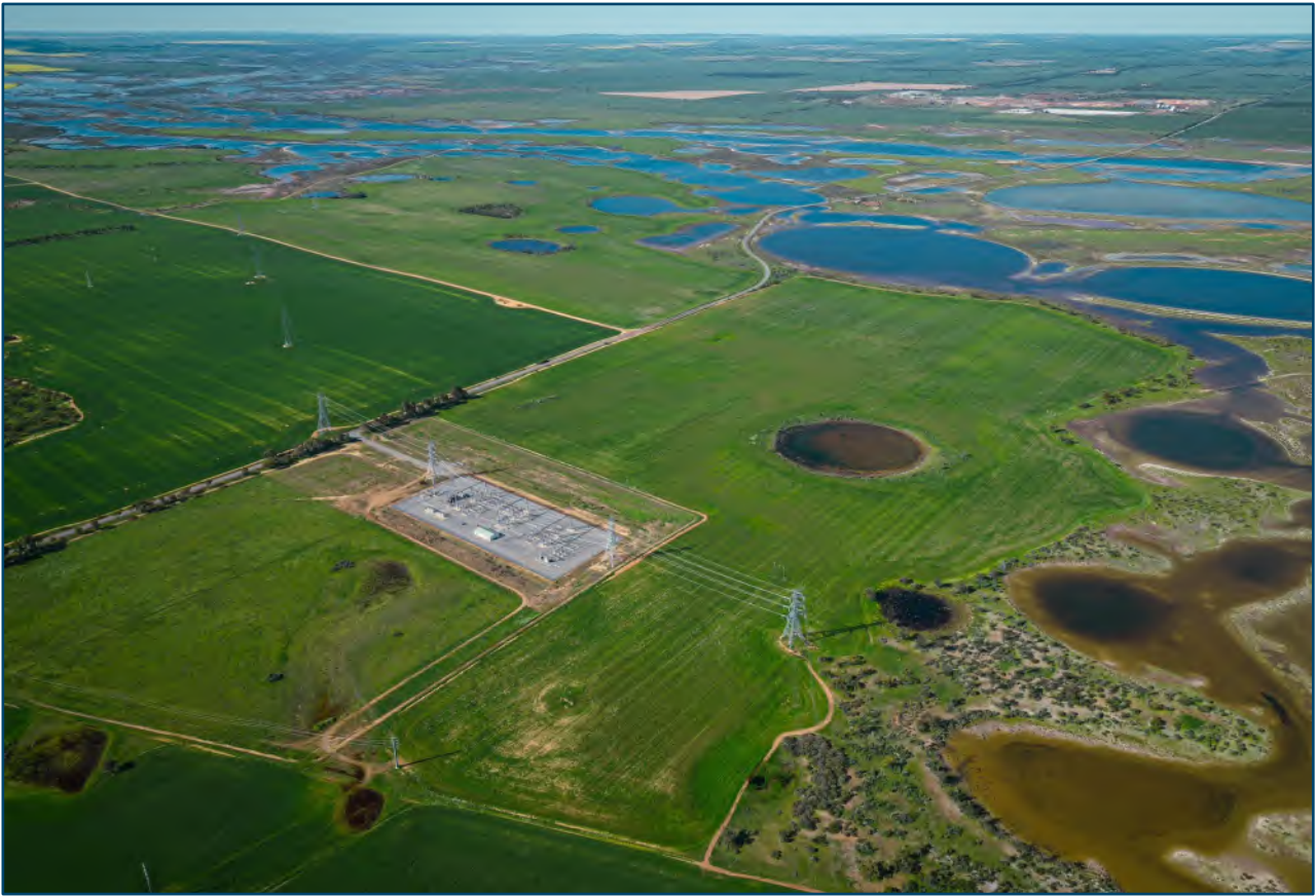
Figure 7 – Drone photograph of the subject site and the Western Power substation (Lot 22), looking north-east.
