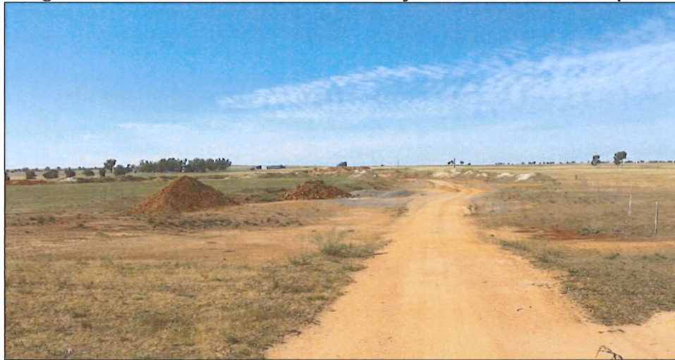
Figure 10.4.7 – View facing west along Skipper Road from western access point
