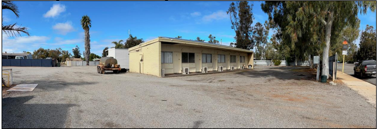
Figure 10.1.8 – View looking south-west from north-east corner
